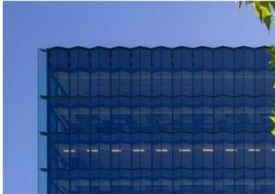
WINDOWS / FRAMING ALUMINIUM FRAMED (UNIVERSAL ANODISERS SATIN CHARCOAL GREY)
